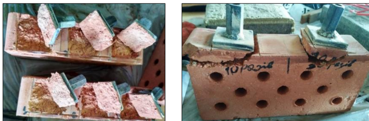
Fig. 5. Torn-off plates with fragments of bricks
